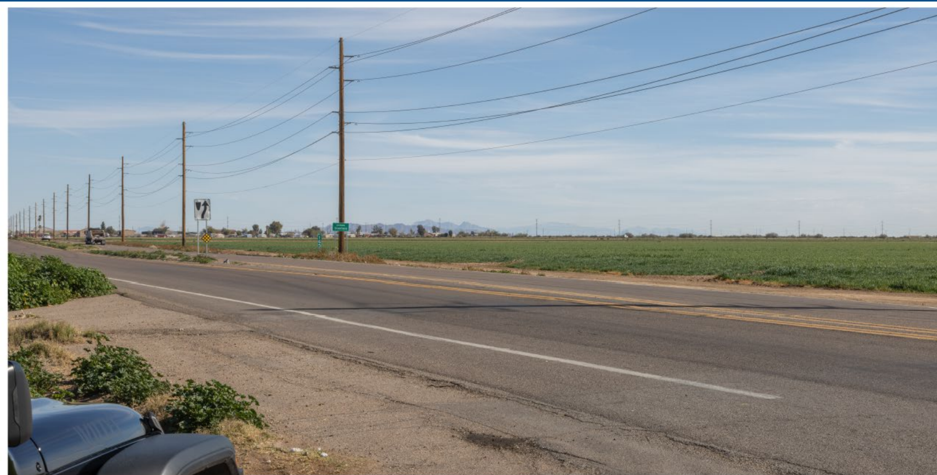
North Fuqua Road & State Route 84 – Looking Southwest
