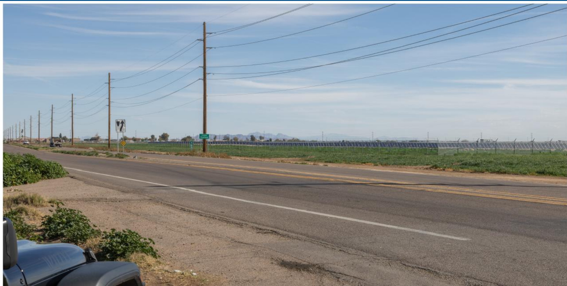
North Fuqua Road & State Route 84 – Looking Southwest
