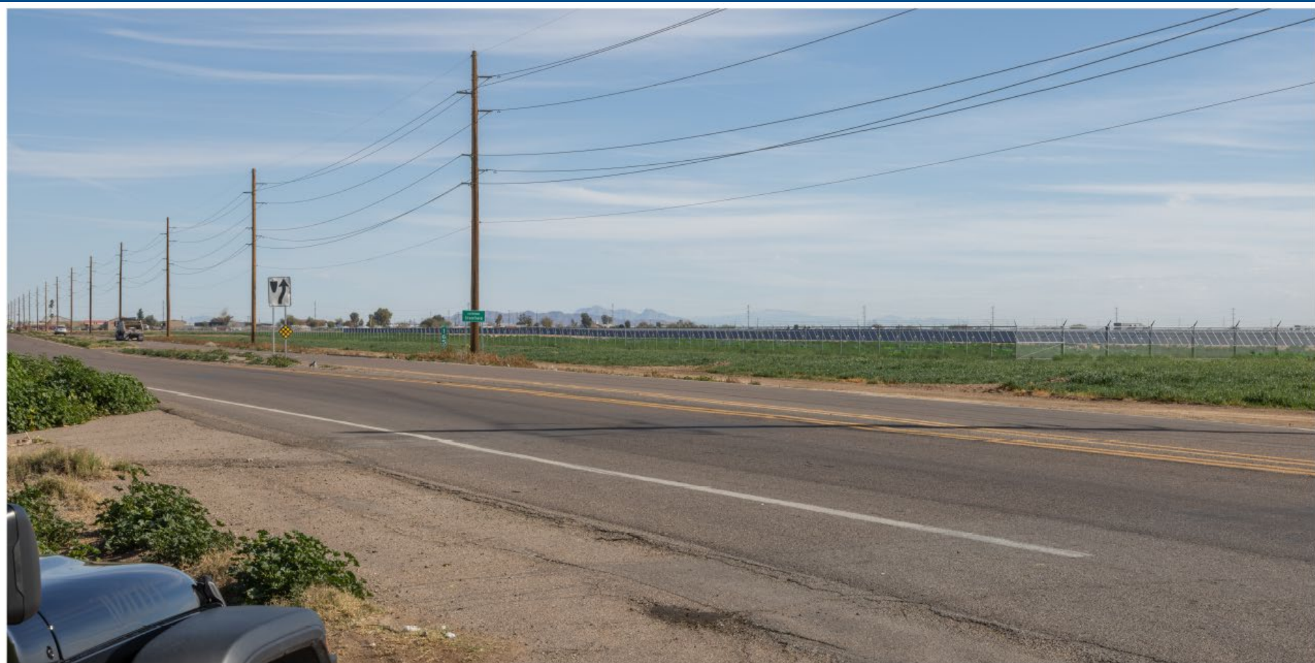
North Fuqua Road & State Route 84 – Looking Southwest
