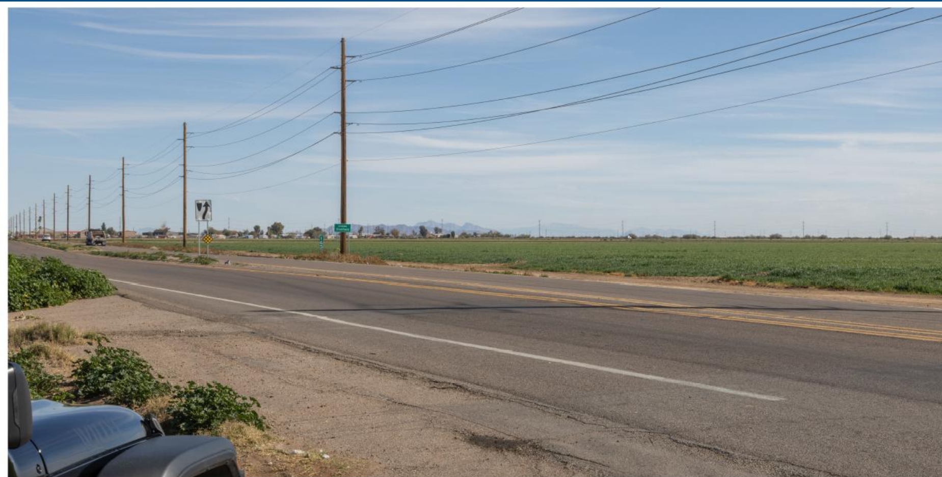
North Fuqua Road & State Route 84 – Looking Southwest
